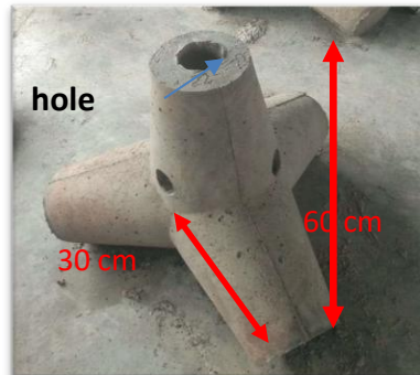
Figure 3. Tetrapods as the foundation of GEHA Apung
